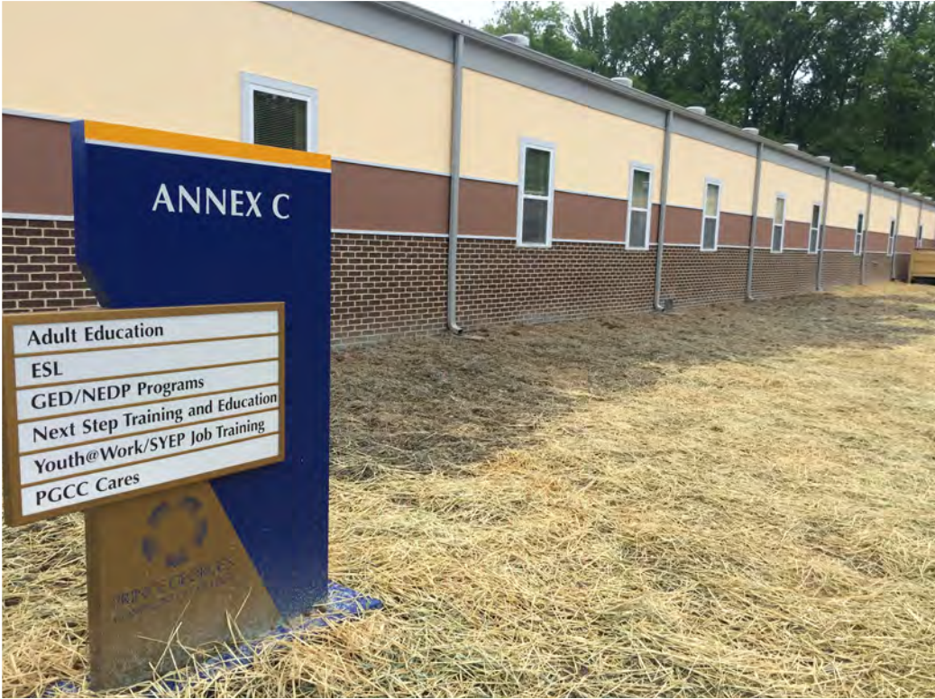
Figure 2.5: Annex C Building
